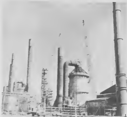
These two cranes are utilized jointly to erect new stack section. Furnace at right, with 150-ft long duct got new insulation lining. E dos gruanan aki ta traha conhuntamente pa instala seccion nobo di e stack. Fomu na drechi, cu su coneccion a haya insulation nobo.
